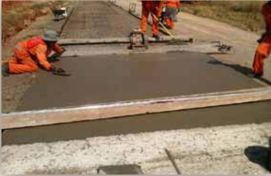
D1264 Concrete Placing and Continuously Reinforced Ultra-Thin Concrete Pavement
