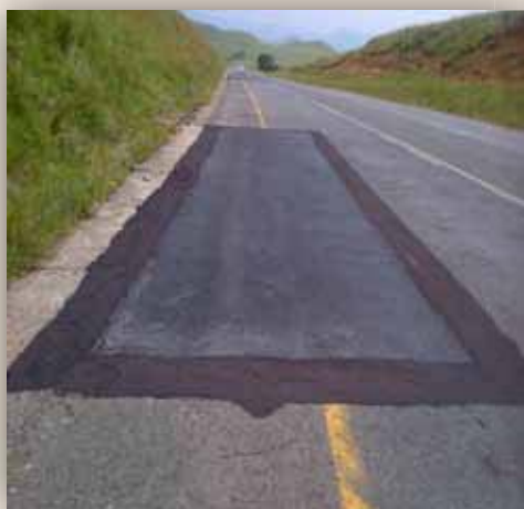
Hlanganani road during and after Black top Patching
