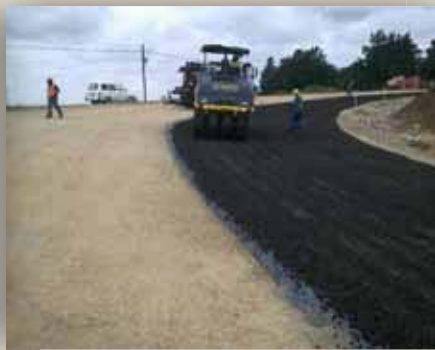
D130/D877 portion of newly surfaced road, P735 19mmstone-1 st seal and P735 after construction
