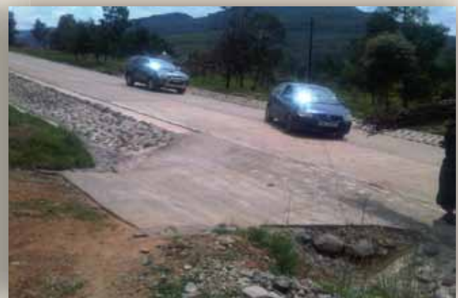
Concrete Stone and Dish Drain
