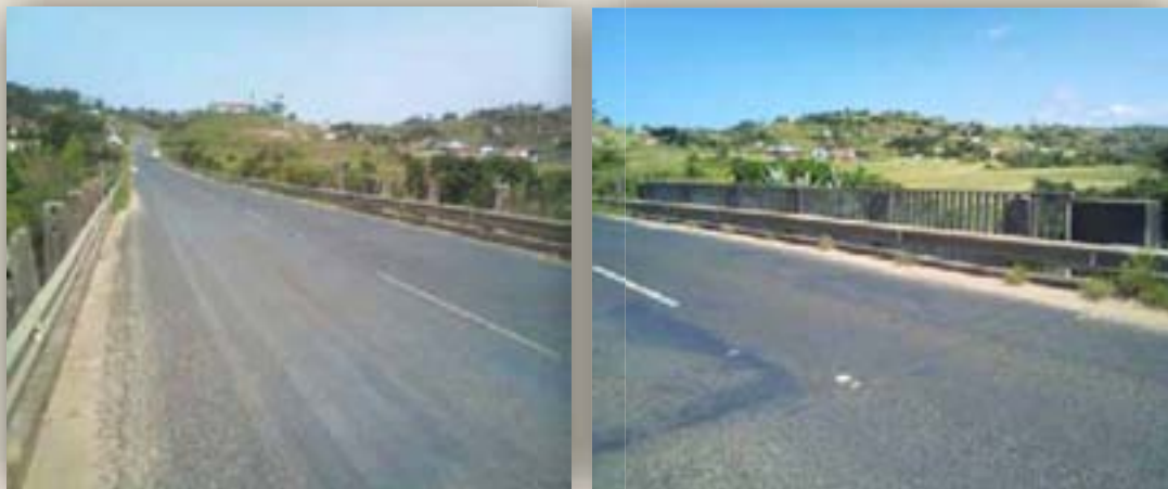
P3-1 before and after Handrail Installation
