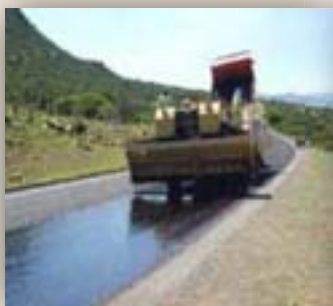
P6-3 reseal in and after progress
