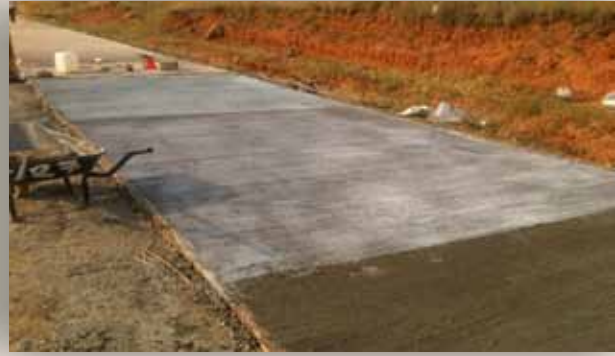
D1264 Concrete Placing and Continuously Reinforced Ultra-Thin Concrete Pavement
