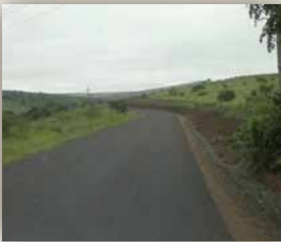
D130/D877 portion of newly surfaced road, P735 19mmstone-1 st seal and P735 after construction
