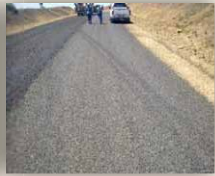
D130/D877 portion of newly surfaced road, P735 19mmstone-1 st seal and P735 after construction
