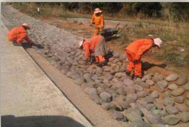
Concrete Stone and Dish Drain
