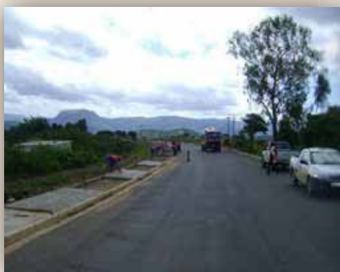
P711 @ km23.8 before, during and after casting of concrete sidewalks
