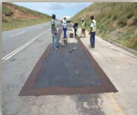
Hlanganani road during and after Black top Patching
