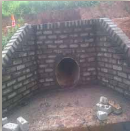
L1954 Ndwedwe Completed Outlet Headwall, with Reno mattress erosion protection and Magwaza Road, Ndwedwe - Construction of Inlet and Outlet Headwall
