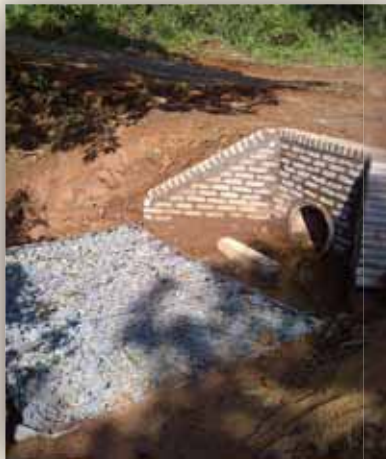
L1954 Ndwedwe Completed Outlet Headwall, with Reno mattress erosion protection and Magwaza Road, Ndwedwe - Construction of Inlet and Outlet Headwall
