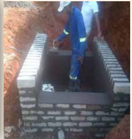
L1954 Ndwedwe Completed Outlet Headwall, with Reno mattress erosion protection and Magwaza Road, Ndwedwe - Construction of Inlet and Outlet Headwall
