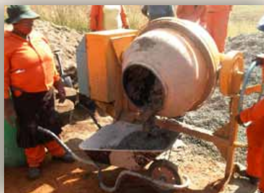
Roadbed Preparation and Concrete Mixing
